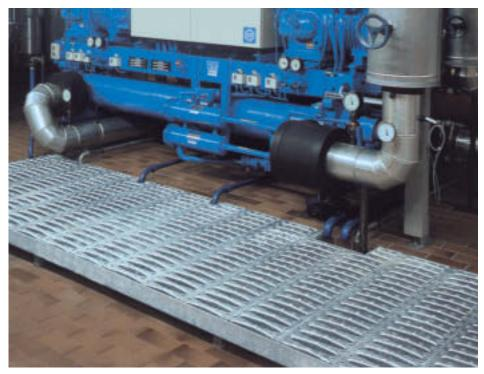
Work platform with perforated metal planks
